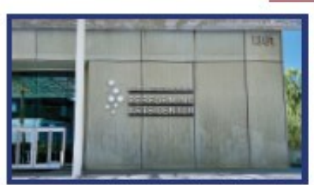
Safe Credit Union Performing Arts Center
